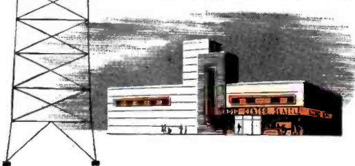
This new FM and television antenna, planned for KOMO, will be the highest structure in the Seattle area, towering 627 feet above sea level.
